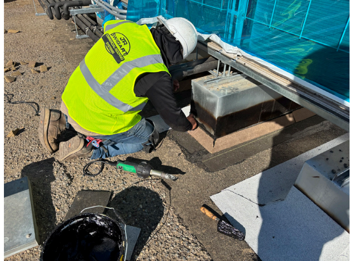
JR Swigert working on the ballasted roof above Evaluation & Treatment.
