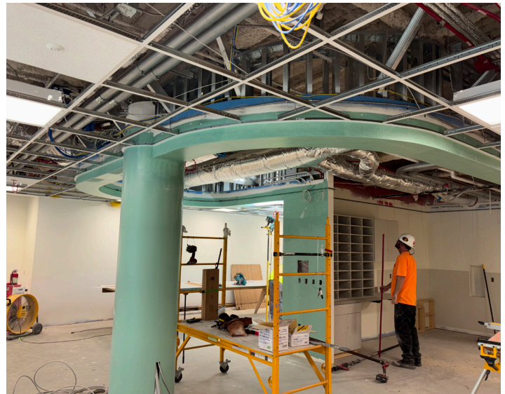
DSI installing ceiling grid for the 9 wood ceilings in Crisis Stabilization.
