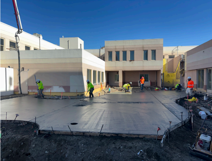
Total Site Services pouring the central courtyard patio.
