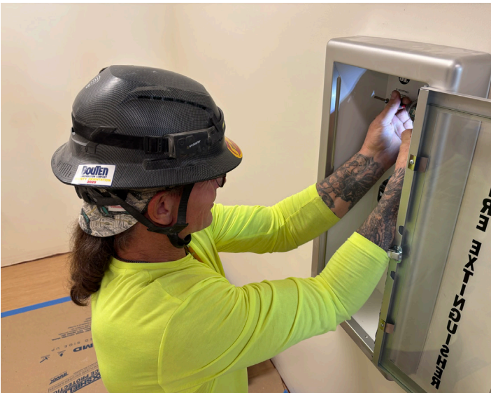
Bouten Construction installing fire extinguisher cabinets throughout Assessment & Exam.
